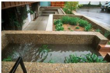
Rainwater collected in planter box then channeled into rain garden Boulder, CO
