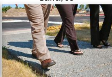
Pervious pavement sidewalk Sioux City, SD
