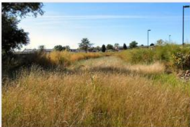
Vegetative swale Fort Carson, CO
