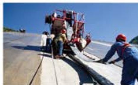
Mechanized Installation of GB Waterstop Materials
