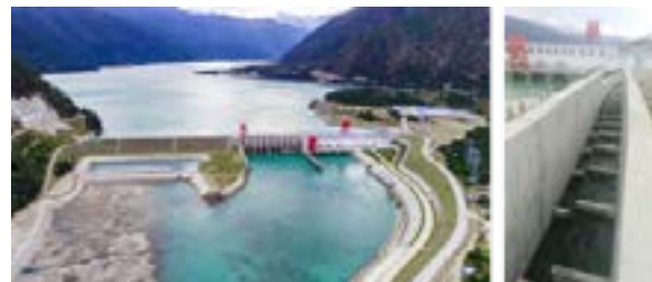
Fishway of Duobu Hydropower Station on Niyang River, Completed in 2016
