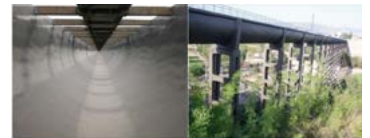
Effect of Internal and External Repair of Aqueduct
