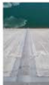
Mechanized Installation of GB Waterstop Materials
