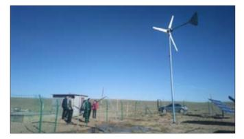
Water supply for the pasture with wind-solar hybrid power system in Inner Mongolia
