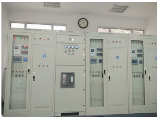
The cabinet housing the low voltage intelligent device units at Shihe Hydropower Station in Qinhuangdao City
