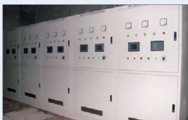
Double micro-computer (PLC) static excitation system for synchronous generator
