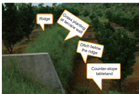
a. Bench terrace with furrow inside and ridge outside plus grass planting at terrace wall
