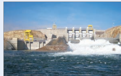
Spillway of Bayramhacili Hydropower Station
